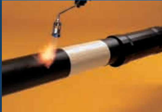
Assembly of insulation half shells.
