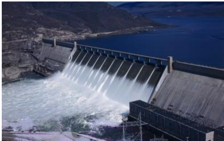
Figure 2. Hydroelectric power plant.
