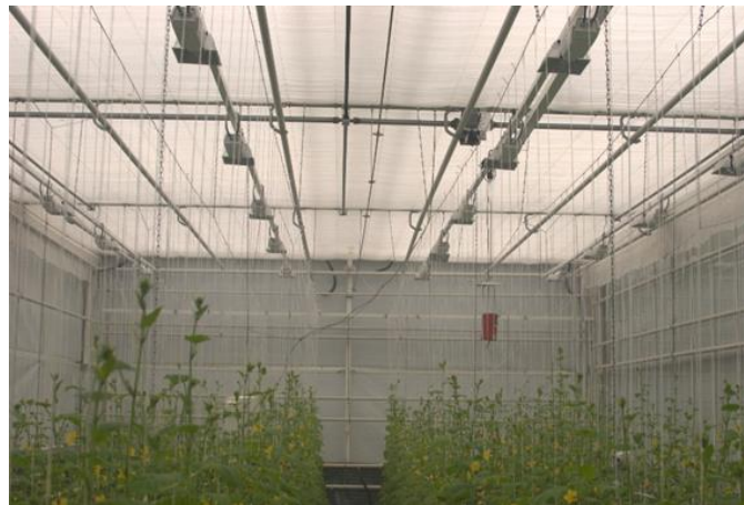
Figure 8. Curtaining system.
