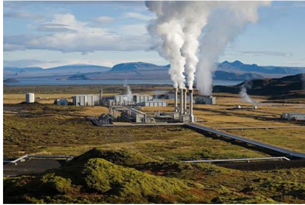
Figure 4. Geothermal power plant.
